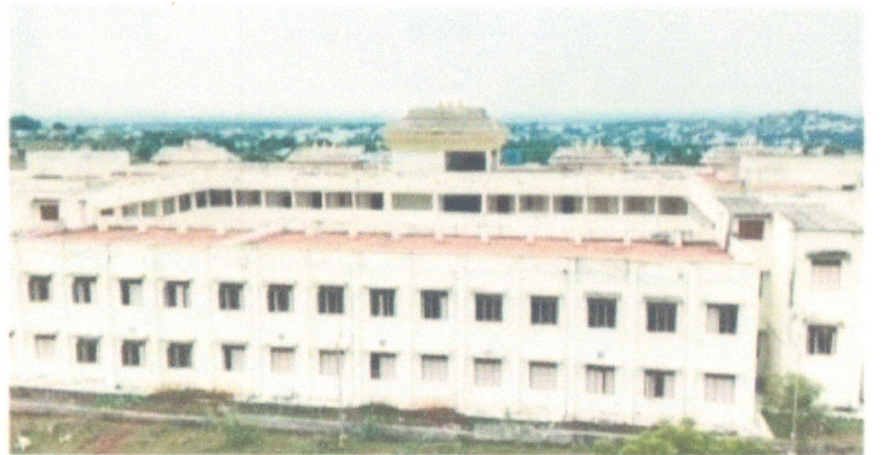
Inside outside View
